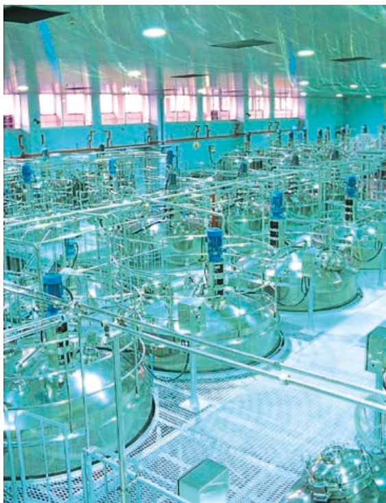
Storage Tanks (Fuji Susono Plant)
