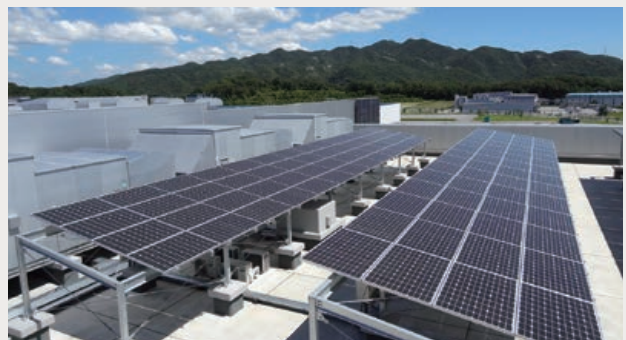
A solar cell electric power generating facility installed on the plant's roof
