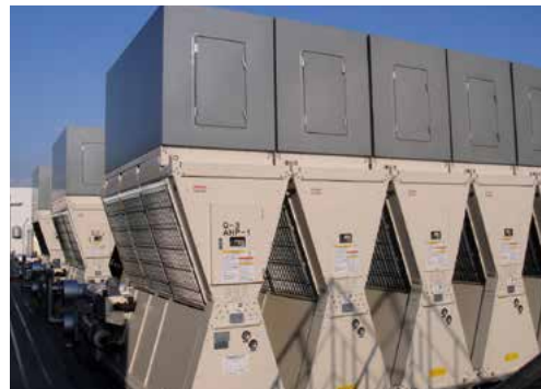
Newly built cool temperature thermal source facilities
