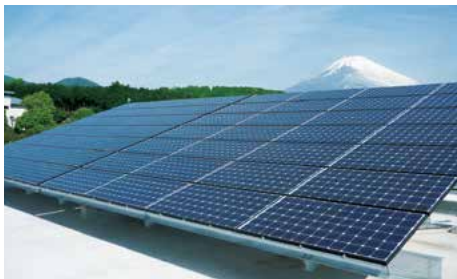
Solar power equipment at the Fuji Susono Plant
