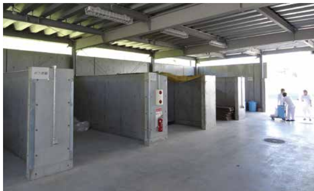
Eco station at the Hyogo Miki Plant
