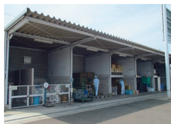
Eco station at Fukushima Plant
