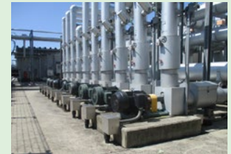
Cooling water pump, Fukushima Plant
