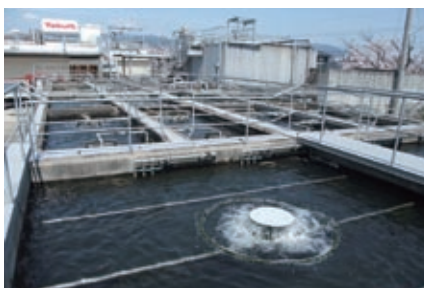
The Saga Plant's Yakult A&G Environmental Water Purification System in operation (This system was being removed as of March 31, 2012, following the plant's creation of a connection to the municipal sewerage system on January 16, 2012.)
