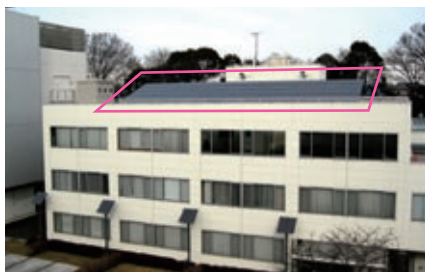
The expanded solar power generation system
