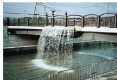
Gake River Heisei-izumibashi Water Treatment Facility, Tokyo
