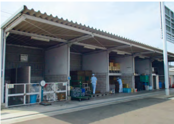
Eco station at Fukushima Plant
